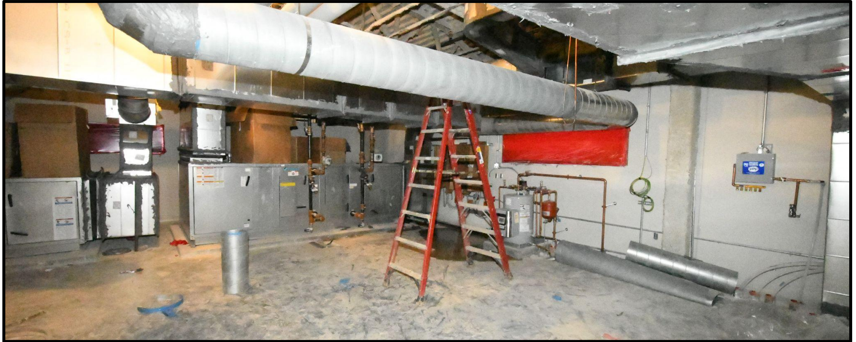
MEP work at Mezzanines
