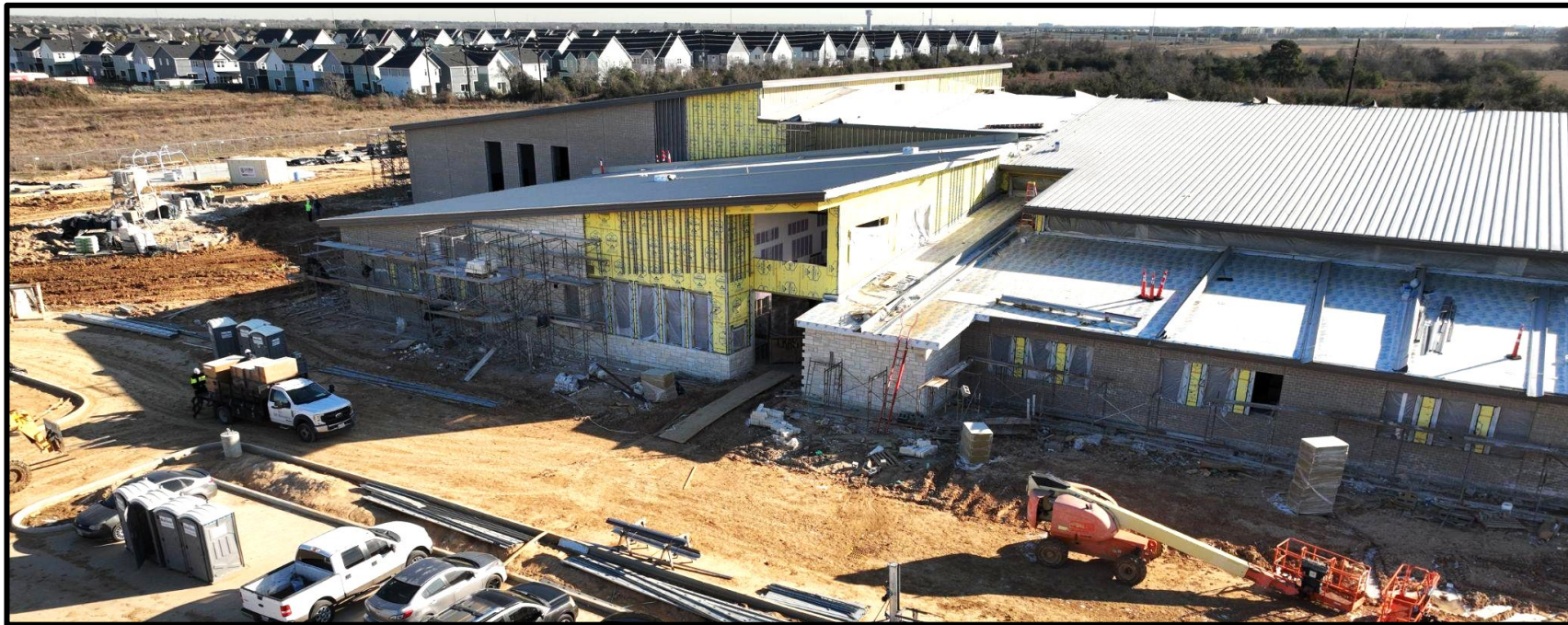
View of Front Entry
