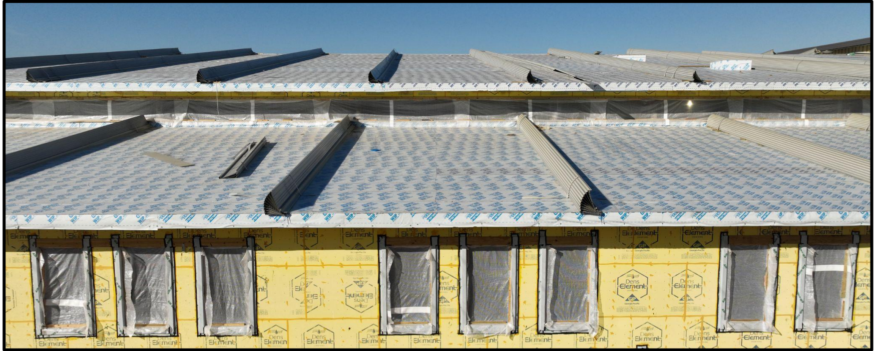
Window Framing in progress
