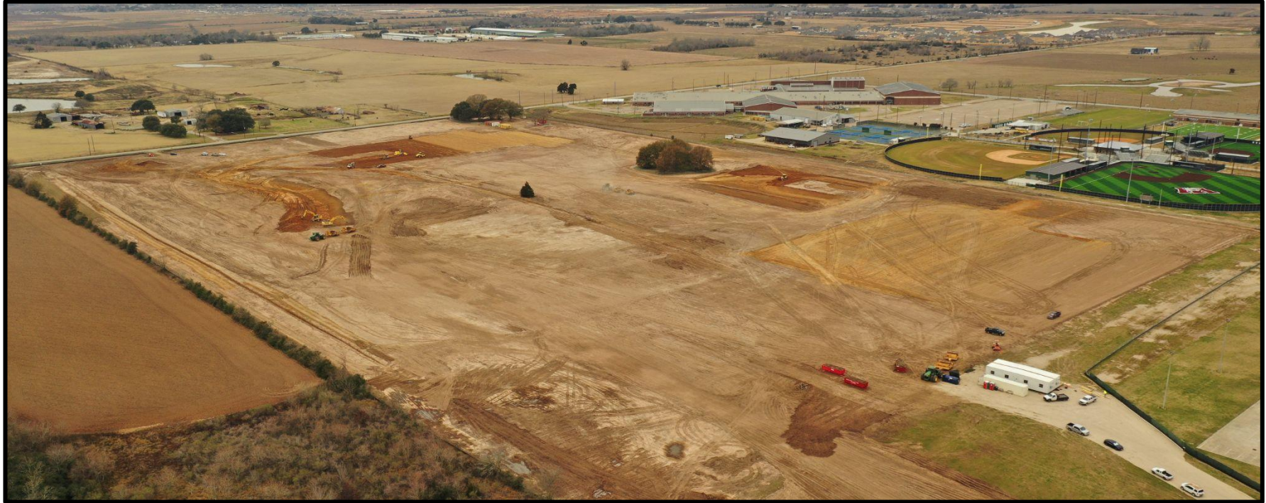
Aerial View - Looking Northwest
